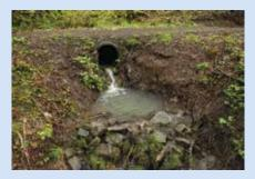
that may accumulate. It is important to grow and maintain a grass covering in the ditches to prevent silt from accumulating and clogging culverts and drainage pipes downstream.
